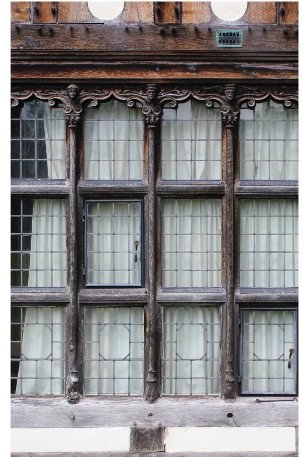
Figure 25 One of the feature windows at Wightwick Manor, highly decorated and with traditional leaded panes.
