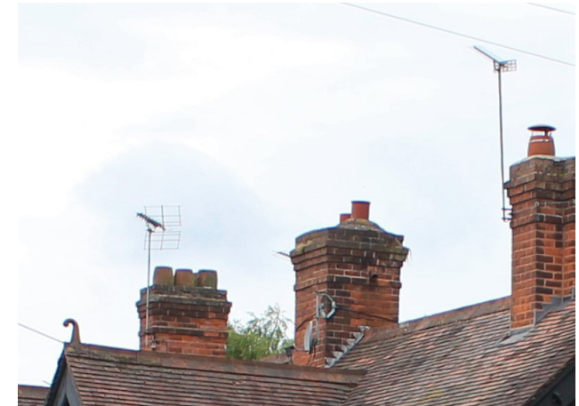
Figure 38 Satellite dishes are visible throughout the Conservation Area. Relocation or removal of dishes is recommended, concealing them from the street scene.
