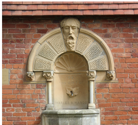
Figure 28 A water fountain, removed from the Market Hall in Wolverhampton, in situ at Wightwick Manor.
