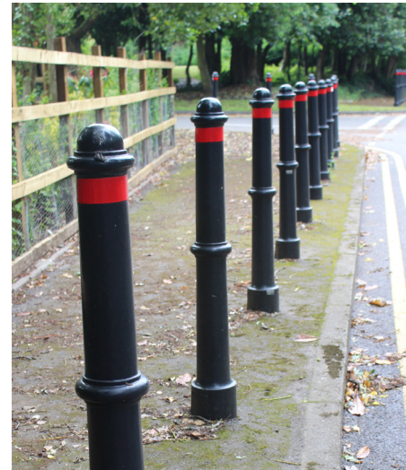
Figure 40 Unsympathetic bollards at the entrance to Elmsdale cul-de-sac.
