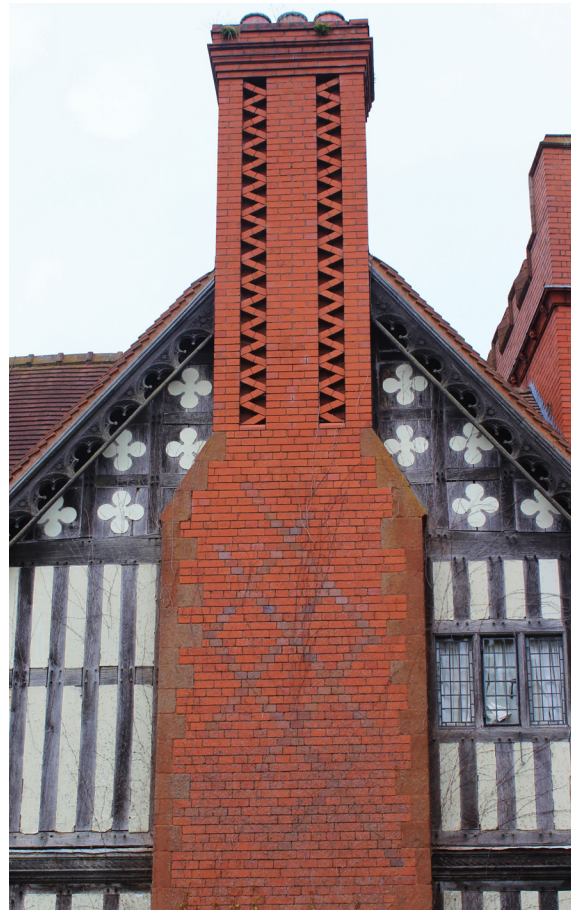
Figure 24 Decorative brickwork, render and exposed timber framing at Wightwick Manor.
