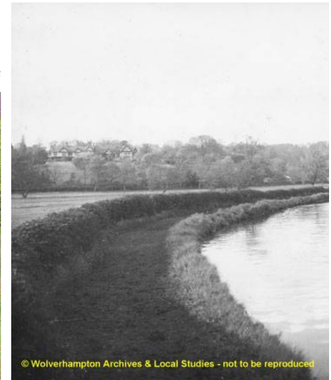
Figure 35 Historic view of Wightwick Manor, viewed from the canal .
